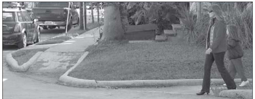
With new curbs pushed back at Willard, the sidewalks no longer meet and pedestrians are forced into the street long before it's safe to cross.
